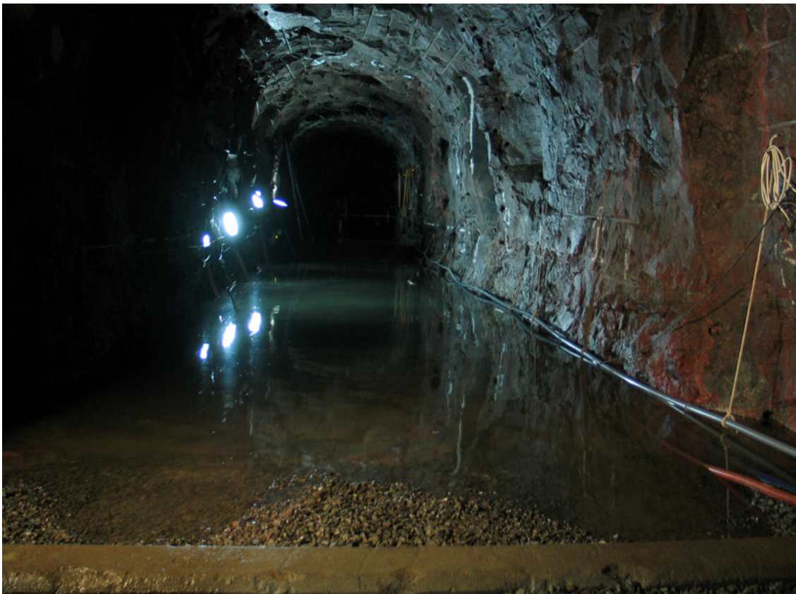
Figure 2-1. Water inflow measurement in the Tass-tunnel, section 0-48.67 m.
