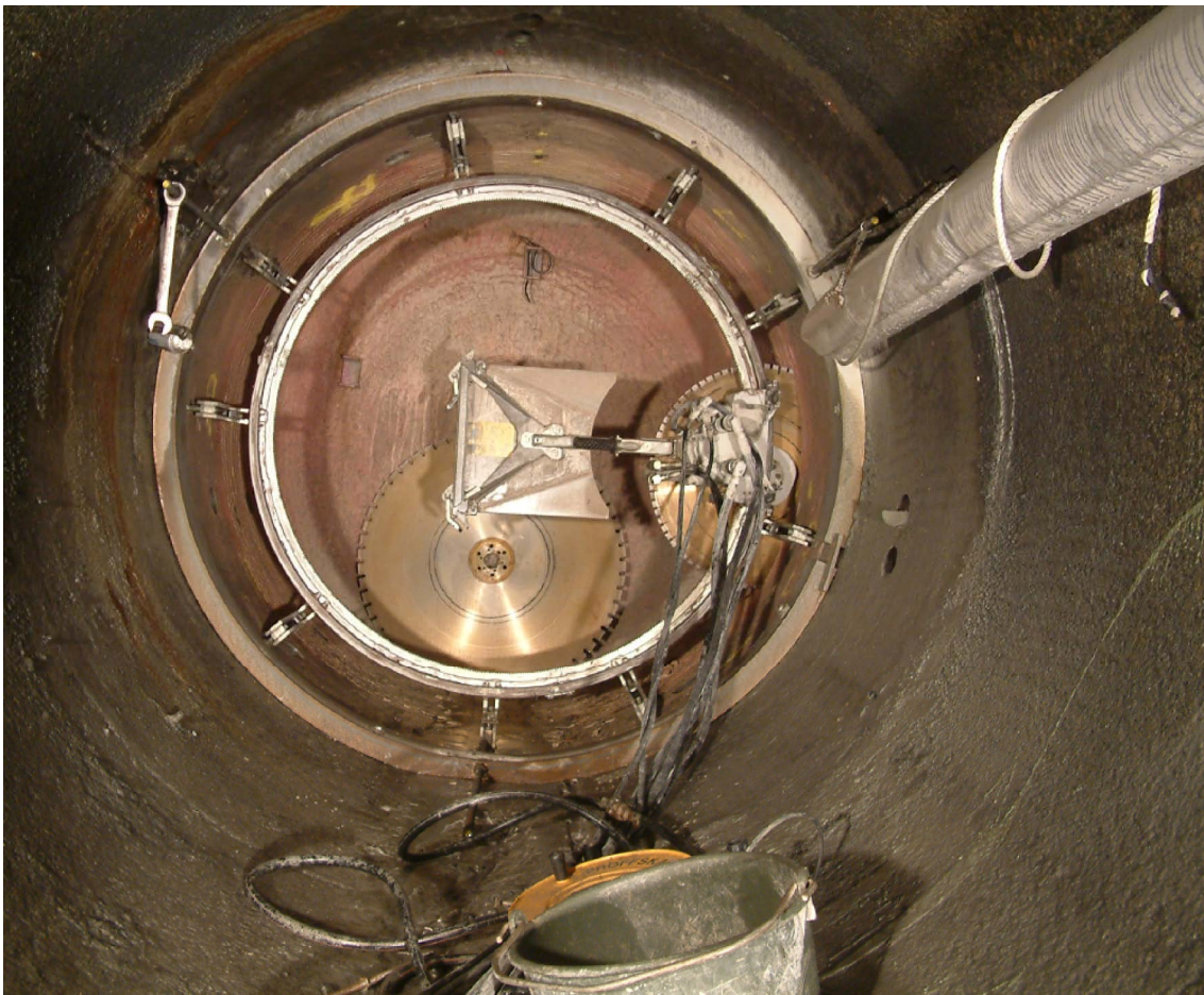
Figure 4-1. KBS-3 Method with Horizontal Emplacement - Excavation of compartment plug rock notch.
